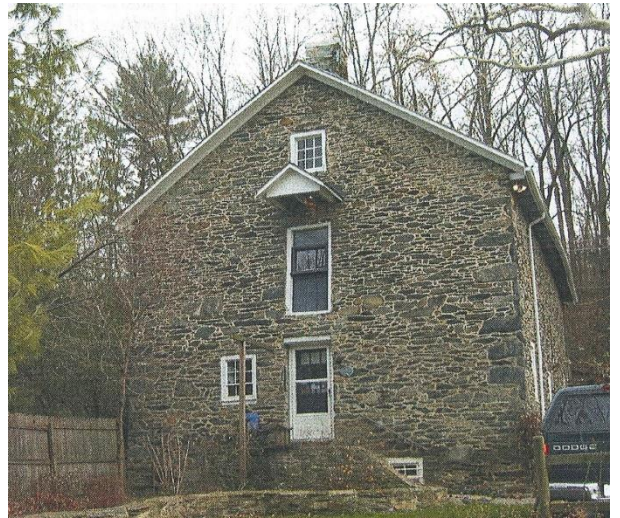
Grubb's Mill ("Thomas Spackman Mill"). Historic Resource #26, photograph from East Bradford Township Historical Commission files
