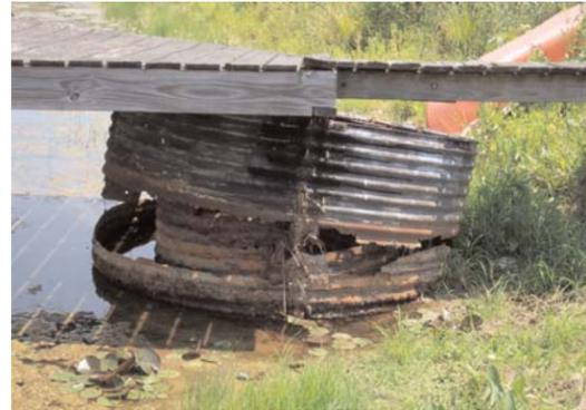
*Standpipes, which control the water level in most ponds, frequently corrode as shown in this photograph. Delaying replacement could result in a more costly expense to the owner of the pond. (Fairchild and Velinsky, 2004)*
