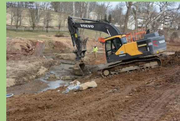
Streambank Regrading and Restoration Process
