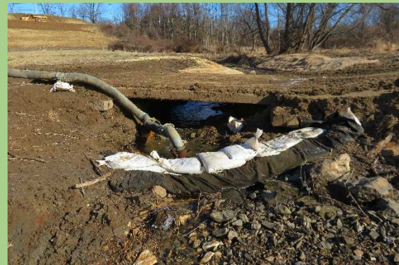
Temporary Stream Diversion
