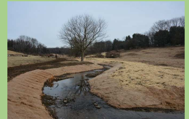
Streambank Stabilization with Single Log Vane Deflector
