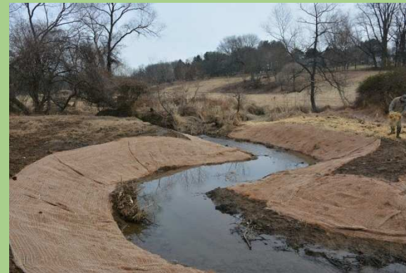
Streambank Stabilization with Root Wad
