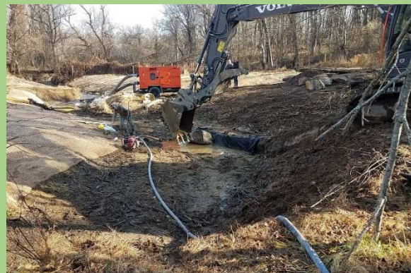
Temporary Stream Diversion
